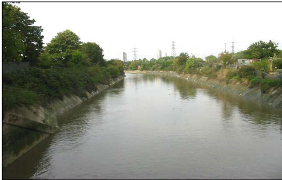
The view northwards up Prescott Channel from the present footbridge. The new lock would stretch 300ft from here and the huge concrete structure would
