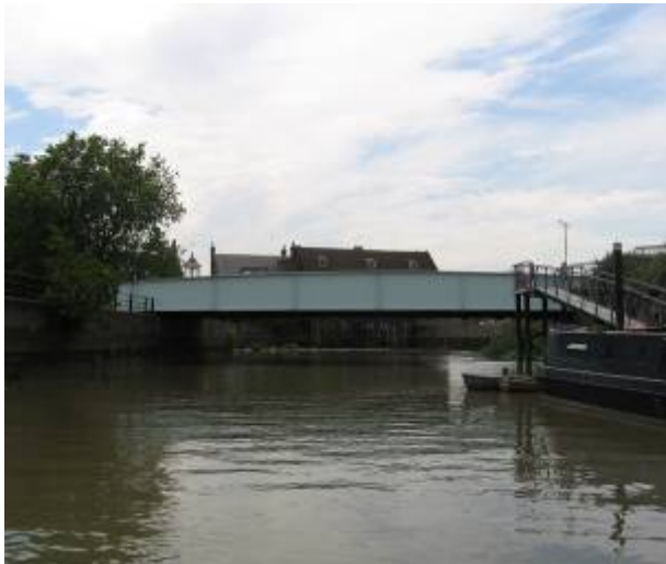
Figure 11 : Looking south towards Three Mills on Three Mills Wall River
