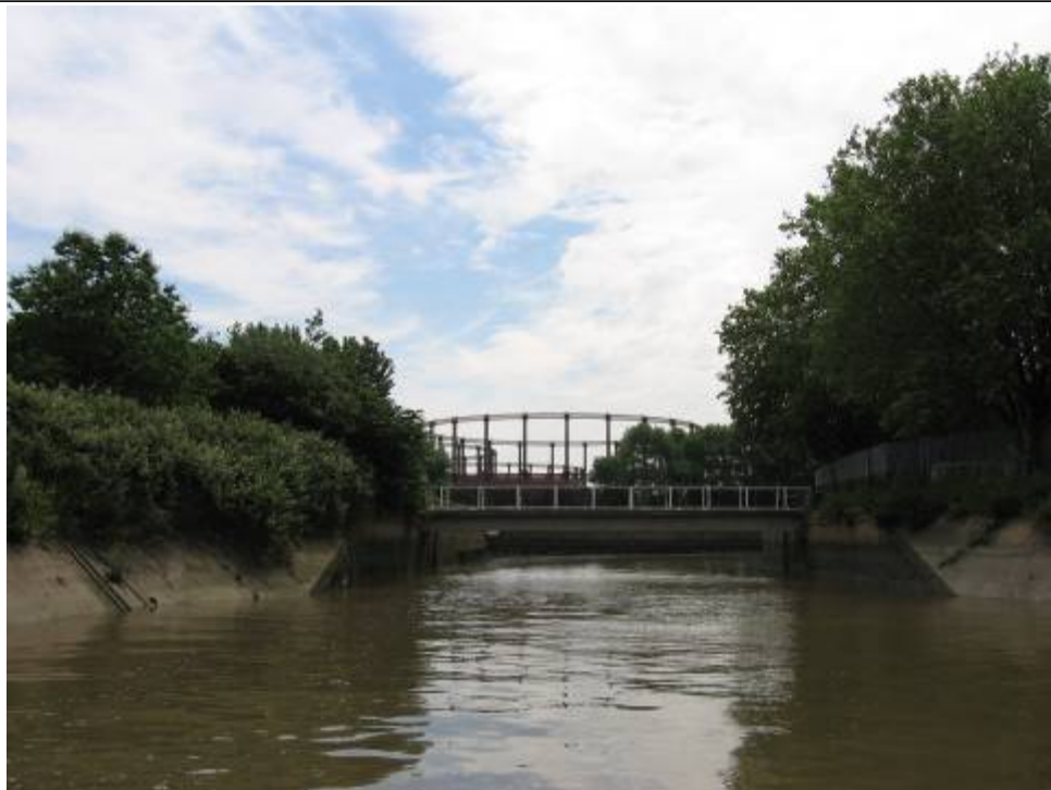
Figure 6 : Prescott Channel looking south at high water
