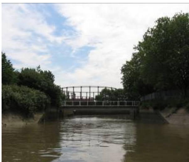
View from Prescott Channel towards Abbey Creek with the listed Gasholders behind
